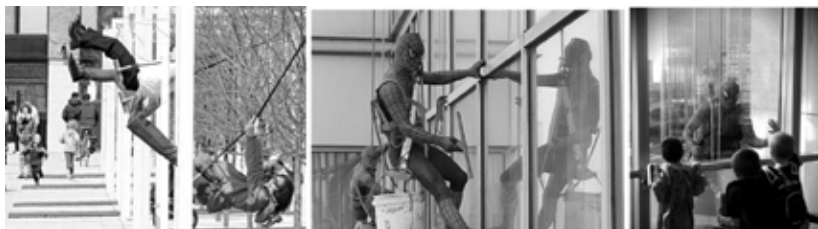
FIGURAS 11, 12, 13 – 21 balançoires e limpadores de janelas do Evelina Children's Hospital
